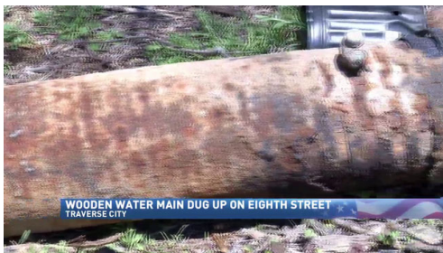
Construction crews found the wooden pipe while digging up Eighth Street this week. (Brittney Buti)
