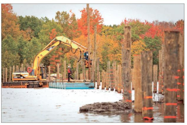
Dave Bale of Team Elmer's works on a barge as posts are driven into Boardman Lake for the boardwalk portion of the Boardman Lake Trail under construction at the lake's south end. The final section of the trail will complete a loop around the lake when completed.
