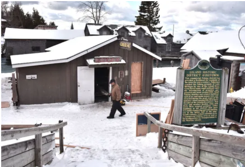
A 1959-built cheese shanty in Leland's Fishtown was reinforced with wood and steel beams prior to it being lifted off its waterlogged and rotting foundation. (Photo: John L. Russell, Special to The Detroit News)
